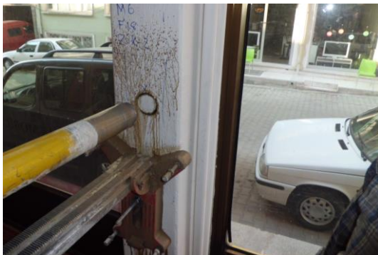
Figure 1. Concrete core sampling from the examined buildings
