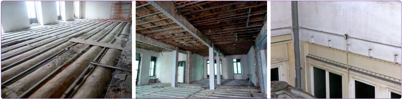
Figure 6. Arched floor system of Pera Palace Hotel.
