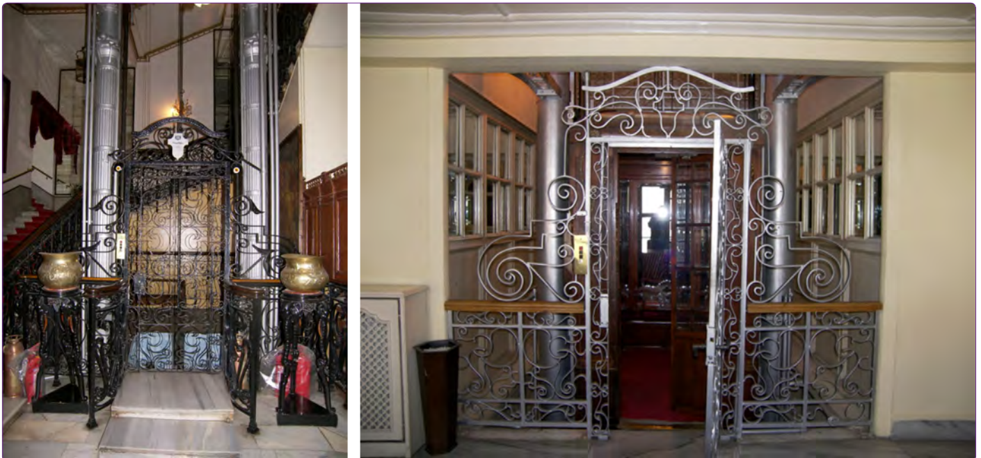
Figure 2. Art nouveau elevator.
