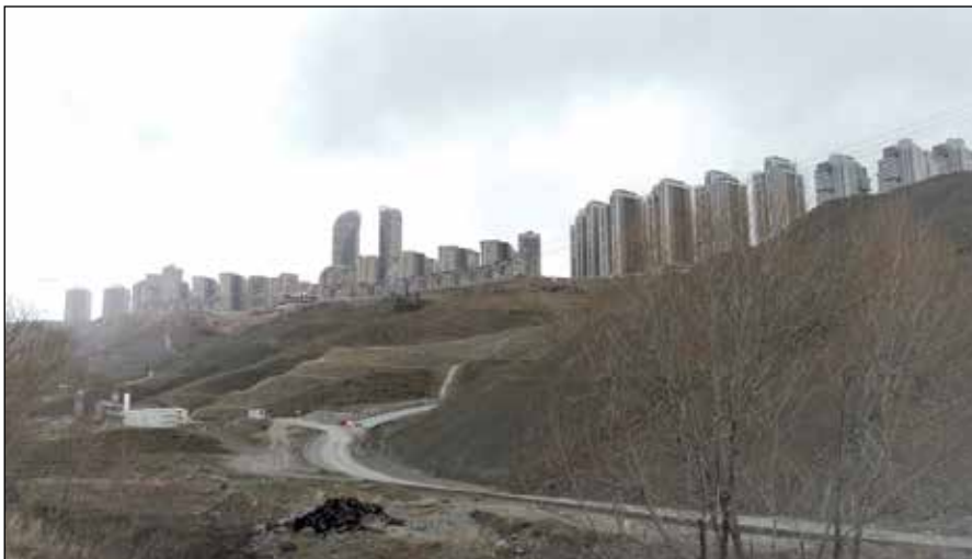
Figure 11. Construction areas in İmrahor Valley.
