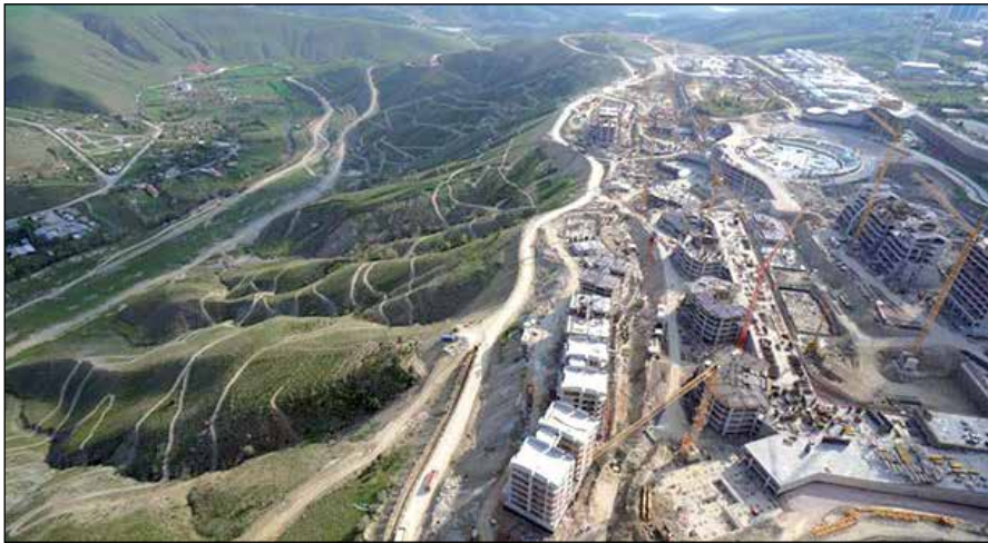
Figure 10. Construction areas in İmrahor Valley.
