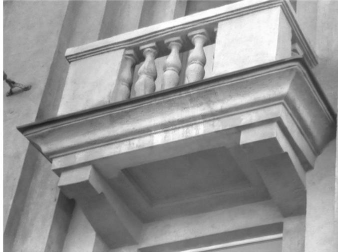
*Figure 2. Photo of a balcony console for calculations of transverse bending.*
