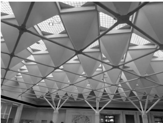
**Figure 5.** Photo of envelopments and frameworks for calculations of combined strength.
