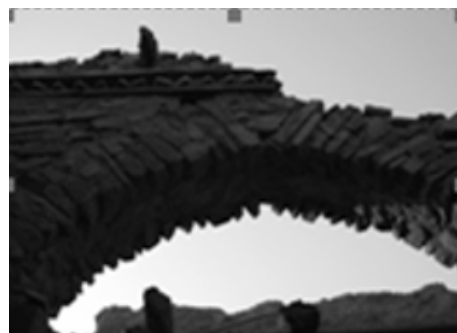
Figure 18. Example of an old arch built according to the constructive tradition of the region: An arcade of the Ksar of KENADZA; Despite the deterioration of the roof and the degradation of the plaster and some stones constituting the arch, the work still resists due to the good disposition of the stones arch built without formwork by flat stones to note the way in which the arc is closed. Source: The culture house wilaya of Bechar.
