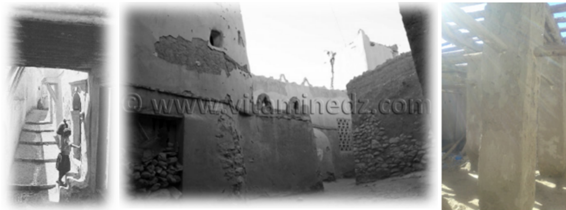
Figure 11. Photo shows the compactness, an example of a lane in a Vernacular popular fabric overlapping floors for shade in the streets and protecting facades of solar rays. Source: https://www.google.fr/search?q=ksar+de+béchar
