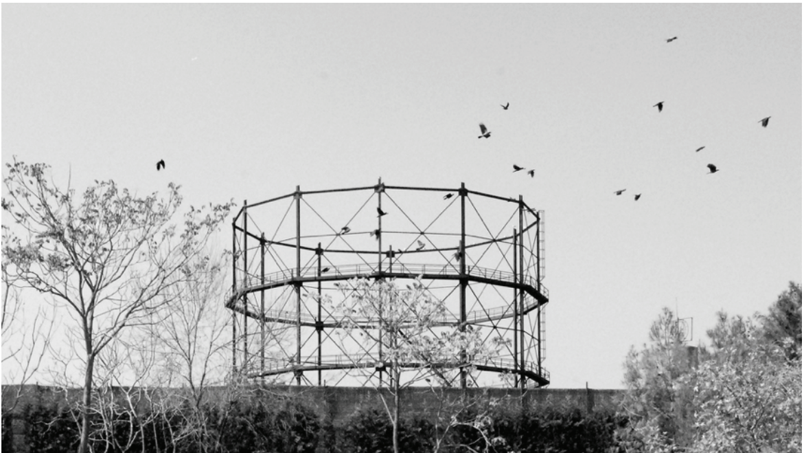
Figure 4. Yedikule Gazometer, 2014, Emre Özdemir.
