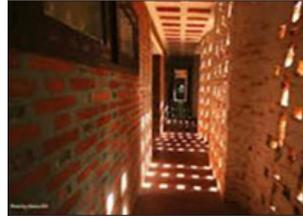
**Figure 35.** Jaali wall provide light and ventilation. (Source:<http://earthbagbuilding.com>).
