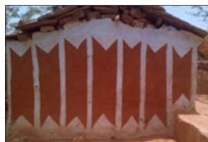
**Figure 21.** The construction of stone wall with mud plaster (Source: Author).
