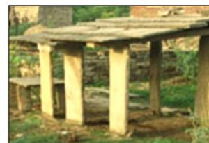
**Figure 23.** The stone roof with the supporting stone members (Source: Author).
