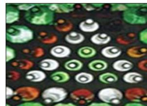
**Figure 43.** The filler slabs made from glass and plastic (Source: <http://insideoutside.in>).
