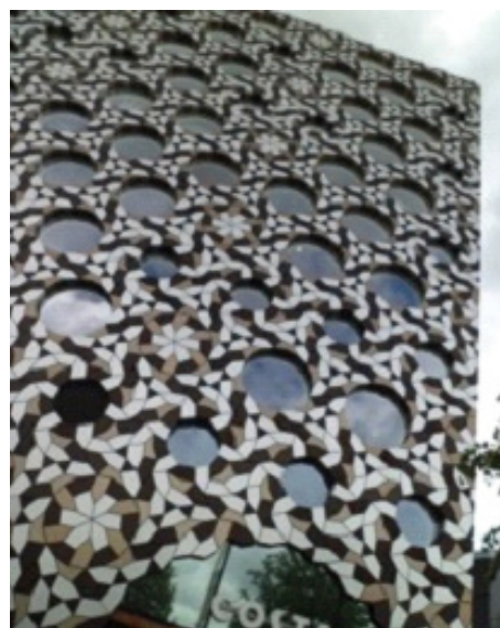
Figure 3. Façade detail of the Ravensbourne College, Foreign Office Architects (FOA), London, UK, 2010.
