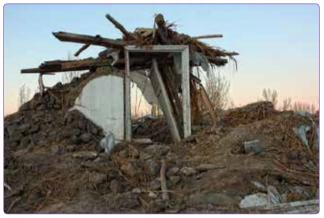
**Figure 4.** A structure with stone walls, broken down as a result of use of undressed stone and low quality mortar (Parsa, A.R. Archive, 2011).
