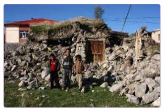
Figure 10. A heavily damaged building with mud ceiling (Parsa, A.R. Archive, 2011).
