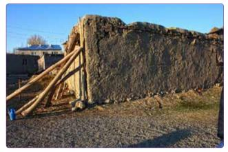
Figure 8. Building which was supported by props after 2011 Van Earthquake (Parsa, A.R. Archive, 2011).
