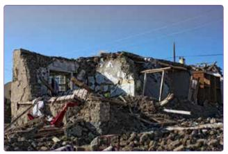
**Figure 3.** An adobe structure damaged by earthquake as a result of inappropriate material choice (Parsa, A.R. Archive, 2011).
